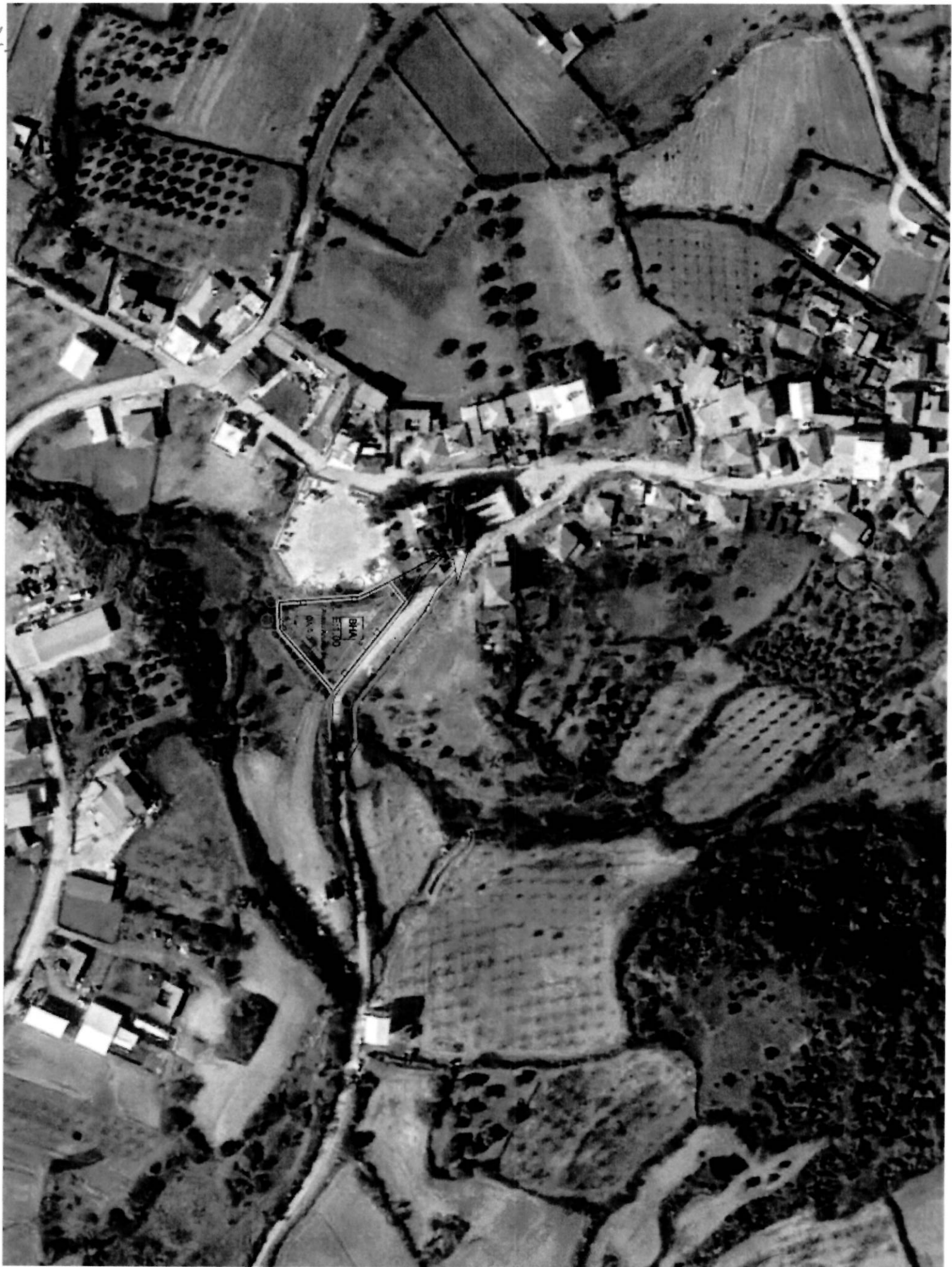
at the edge of the road
